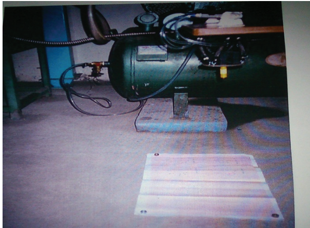
Fig Assembly of Stewart platform using Air muscle with Compressor
