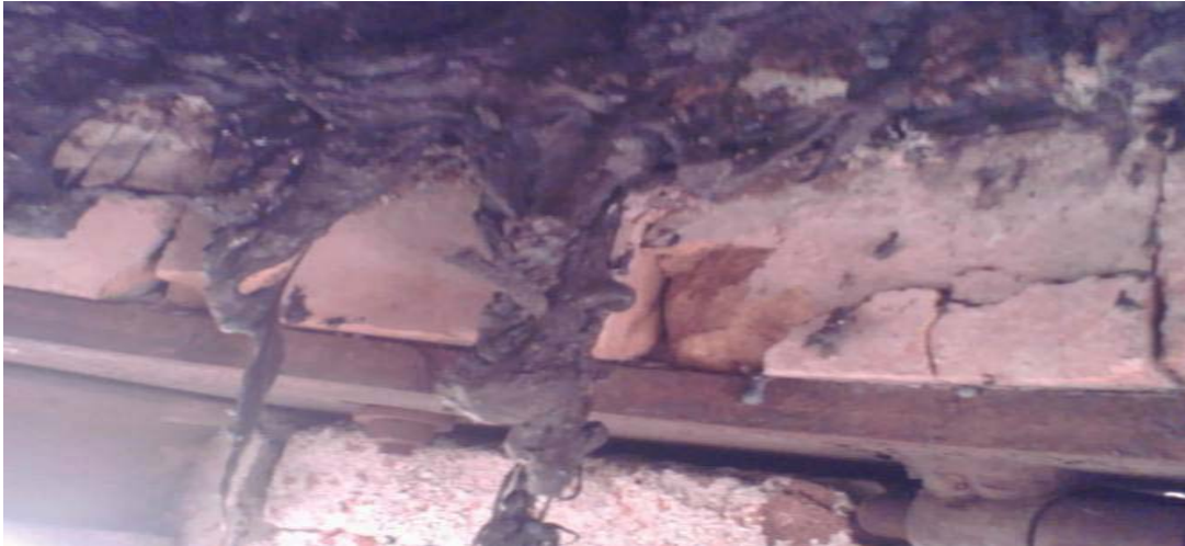
Figure-1. Spent fire brick in kiln operation
