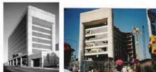
Figure 1-1 Alfred P. Murrah Federal Building Before and after Explosion
