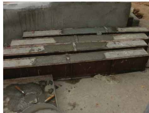
Application of repair materials
