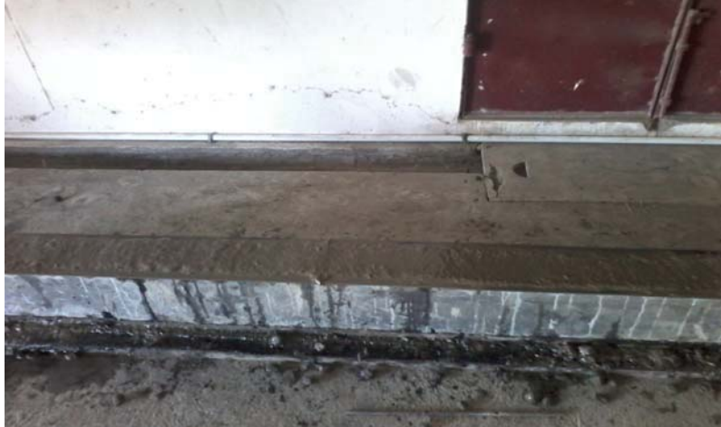
Figure 3. Casting Of Beam And Surface Finishing
