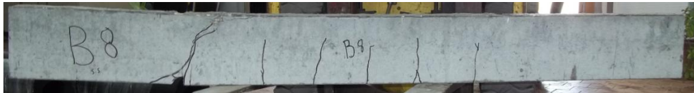
Figure 20. Crack Pattern of Beams B8
