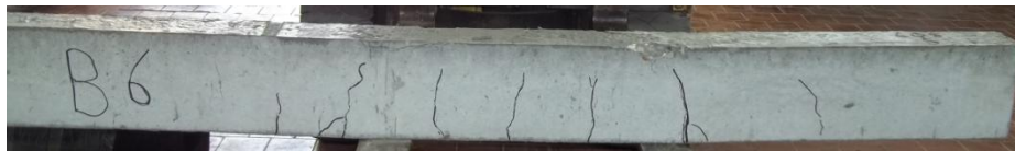
Figure 17. Crack Pattern of Beams B6
