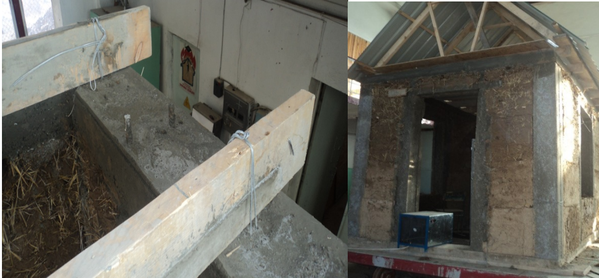
Fig 5. The process of construction of model homes from the «reinforced concrete frame»
